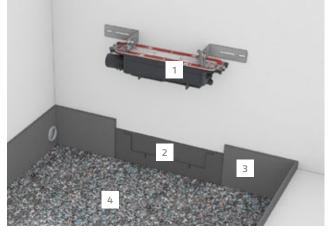
Step 1: Before the drain is inserted, the shower area is expertly prepared by installing the sound insulation strip, the edge insulation strip and a sound insulation mat for impact sound insulation.
