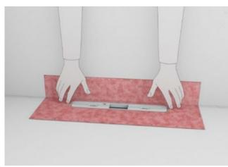
Step 4: Sealed with a click: once the screed has been installed, the first part of the bare-wall protection is removed from the drain and the sealing sleeve supplied is inserted via the click mechanism. The shower area can now be sealed and tiled.
