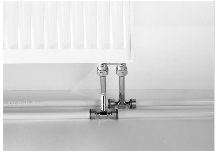
Radiator connection with radiator mounting tee
