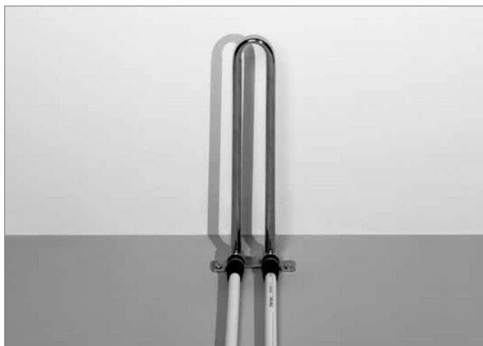
Radiator connection with radiator mounting unit, floor-mounting - ready for pressure test
