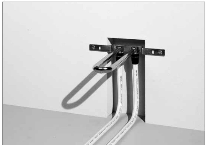
Radiator connection with radiator mounting unit, wall-mounting - ready for pressure test
