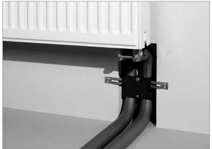
Radiator connection with mounting module - connected to the valve block
