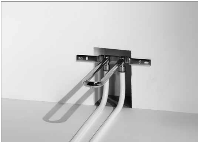
Radiator connection with radiator mounting unit - ready for pressure test
