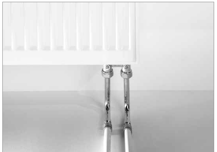
Radiator connection with radiator mounting elbow
