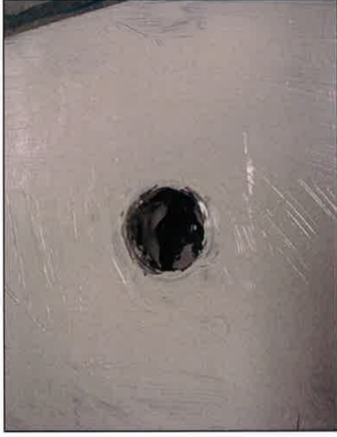
Fig. 3.3: Test specimen – water inlet WC pan
