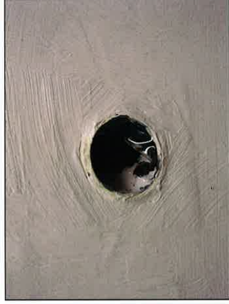
Fig. 4.2: Test specimen – water inlet WC pan
