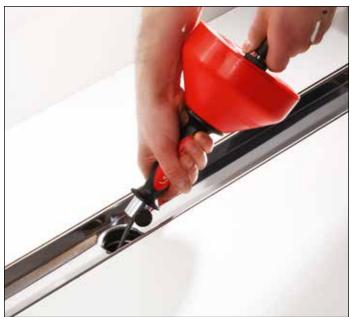
Clean the outlet pipe with a small manual pipe cleaning cable
