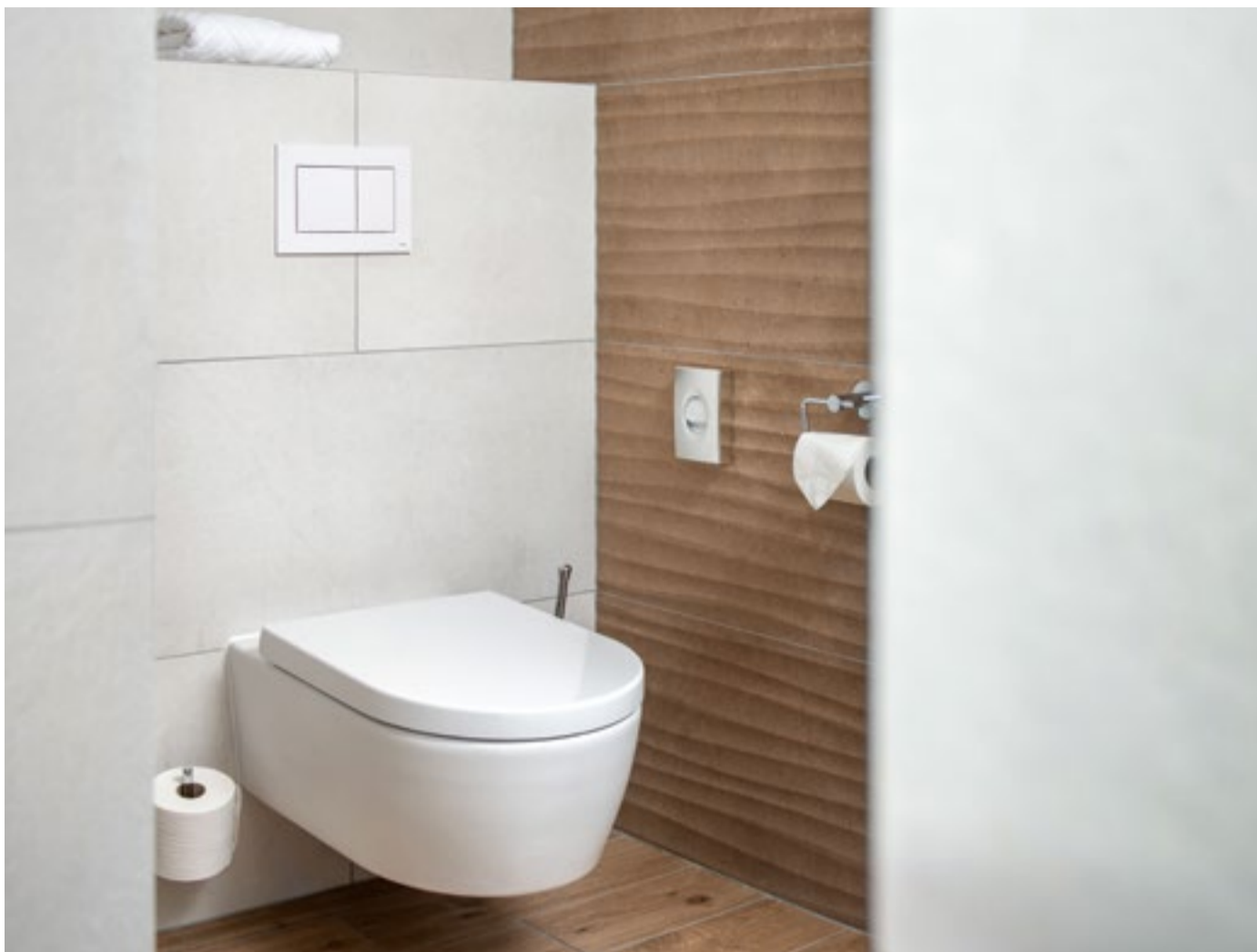
The bathrooms of the Hilton Garden Inn Hotel were completed quickly and efficiently with prefabricated TECESystem sanitary walls.
