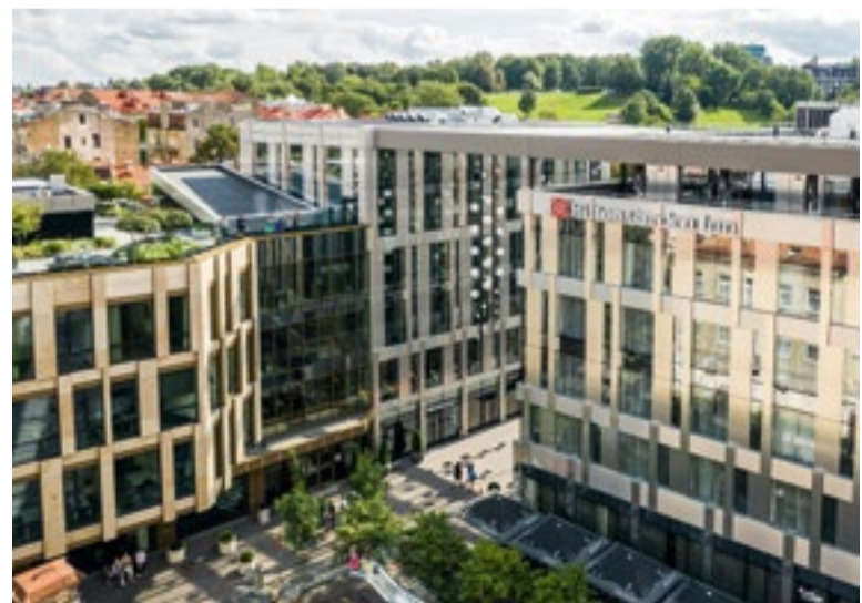
The Hilton Garden Inn Hotel project in Vilnius was the first time that prefabricated TECESystem sanitary walls had been used in Lithuania to optimise the construction process of a project of this size.
