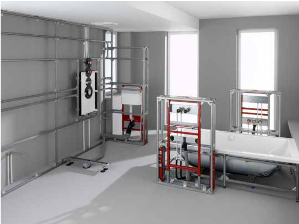
Bathroom walls with TECEprofil – before
