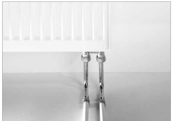
Radiator connection with radiator mounting elbow
