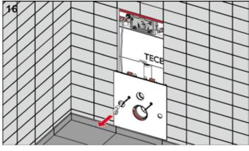
Guide the reinforced hose through the hole provided for the purpose in the glass facing.
