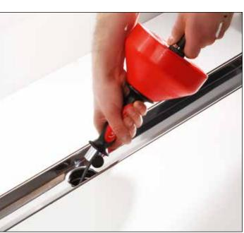
Clean the outlet pipe with a small manual pipe cleaning cable
