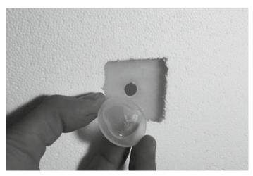
Immediately place the disk on the opening and press lightly. The drying time is approx. 15 minutes. Fill the cistern and check the seal.
