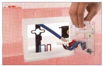
Splash guard with actuation block
