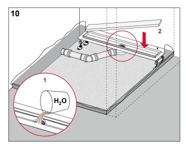
Test for leaks and then place the protective cover back in the channel.
