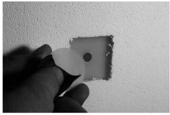
Clean the area to be repaired thoroughly using a solvent or acetone.
