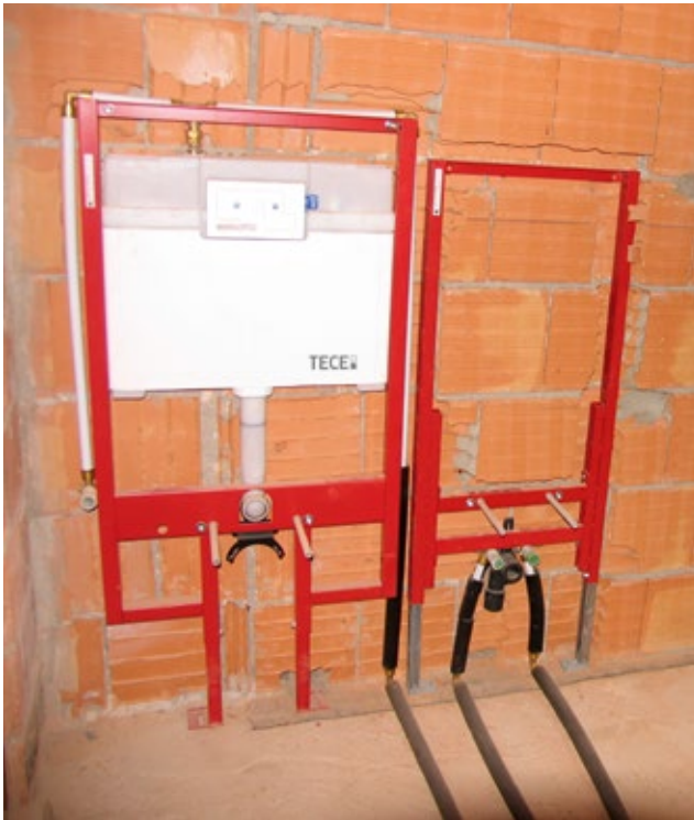
Internal walls in Italy are usually only 8 cm thick. This requires a special cistern with a low installation depth and high level of sound insulation.
