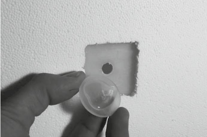
Immediately place the disk on the opening and press lightly. The drying time is approx. 15 minutes. Fill the cistern and check the seal.
