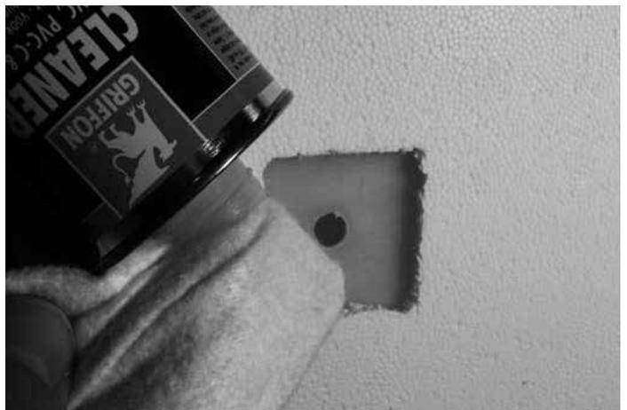
Insert a glue stick into the hot glue gun and apply the glue to the plastic disk (the covered area must be twice as large as the diameter of the opening). Only use the original adhesive and do not mix this with other adhesives!
