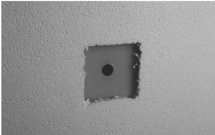
Round off the edges around the opening with a cutter knife.
