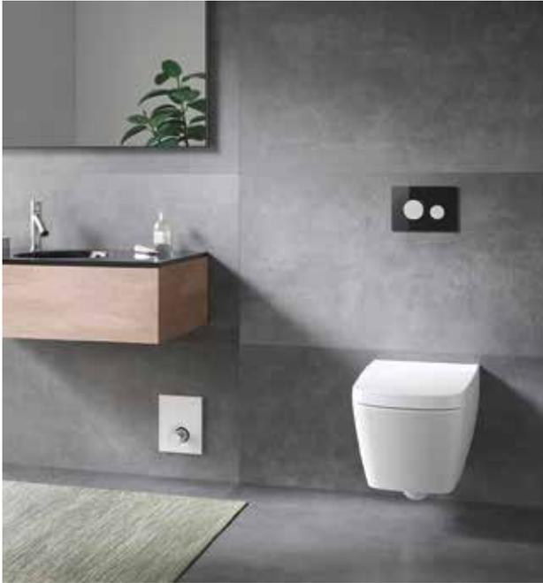
Conventional RTL boxes are relatively large and together with the thermostat head they protrude several centimetres from the wall. They are therefore often placed out of sight, usually near the floor. However, this results in an inaccurate measurement of the room temperature and it is inconvenient to operate.
