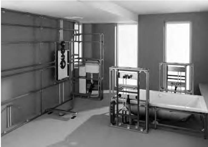
Bathroom walls with TECEprofil – before
