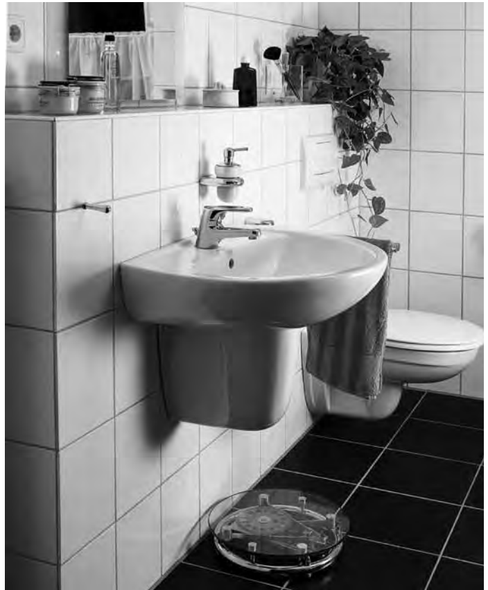
Completed sanitary installation
