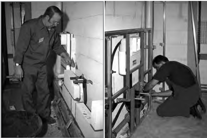
Brick-wall construction(left) compared with dry-wall construction
