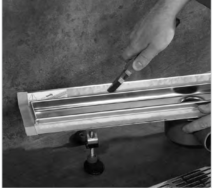
Bending the channel flange
