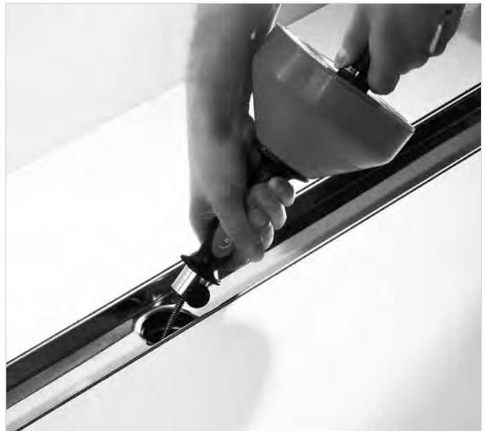
Clean the outlet pipe using a small manual pipe cleaning coil
