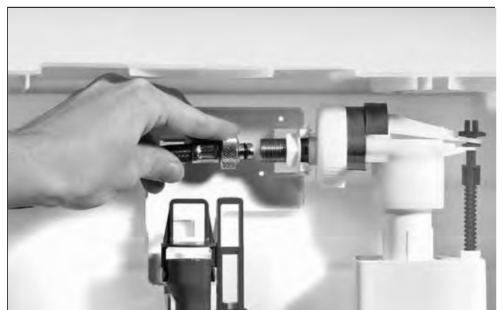
Connection of the armoured hose to the filling valve
