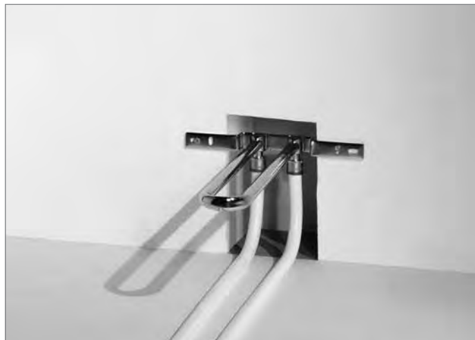
Radiator connection using radiator mounting unit – ready for pressure testing
