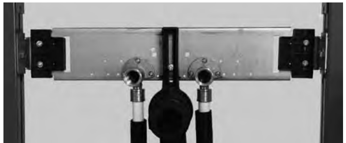
Sound insulation of crossbeam from module frame
