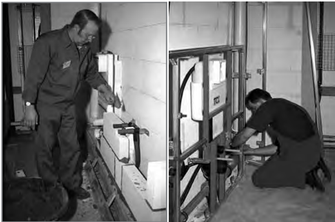
Brick-wall construction(left) compared with dry-wall construction
