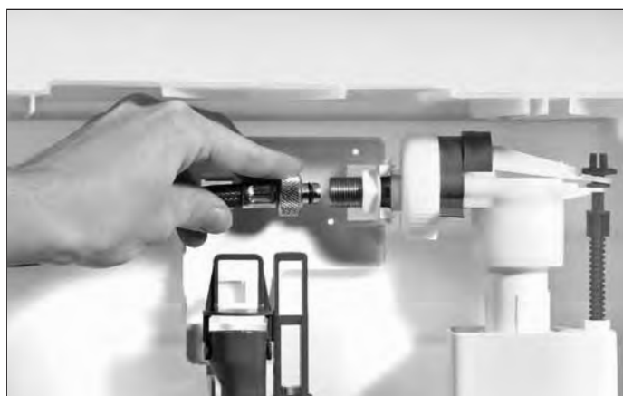
Connection of the armoured hose to the filling valve
