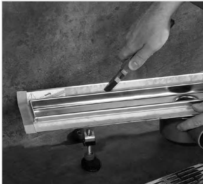
Bending the channel flange
