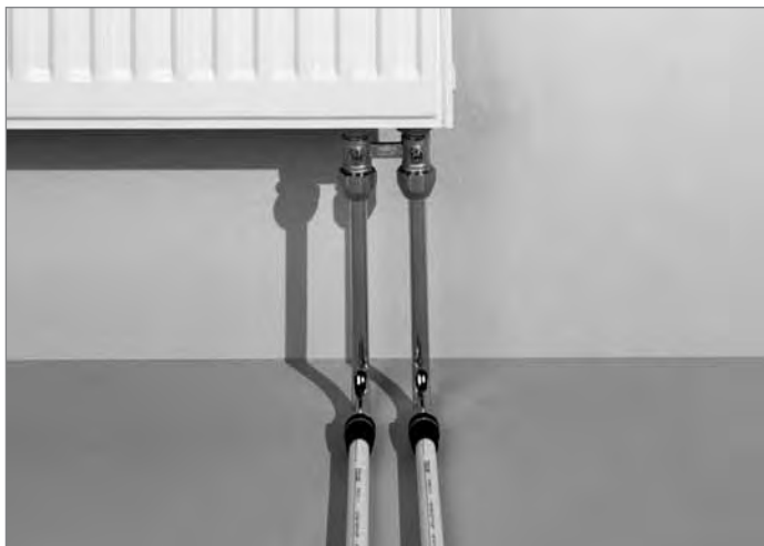
Radiator connection with radiator mounting elbow
