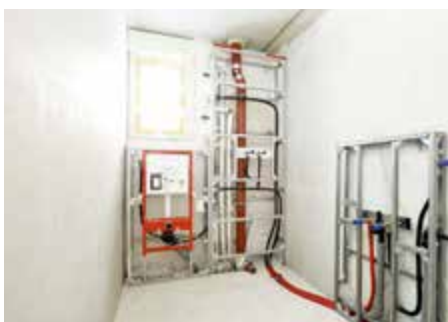
TECEsystem after assembly
